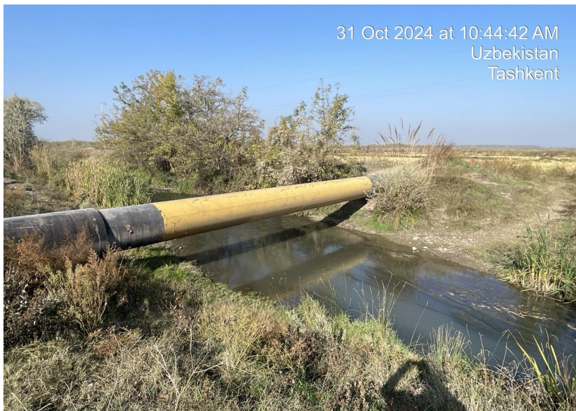
Gas Pipeline to the West of the Project Site
